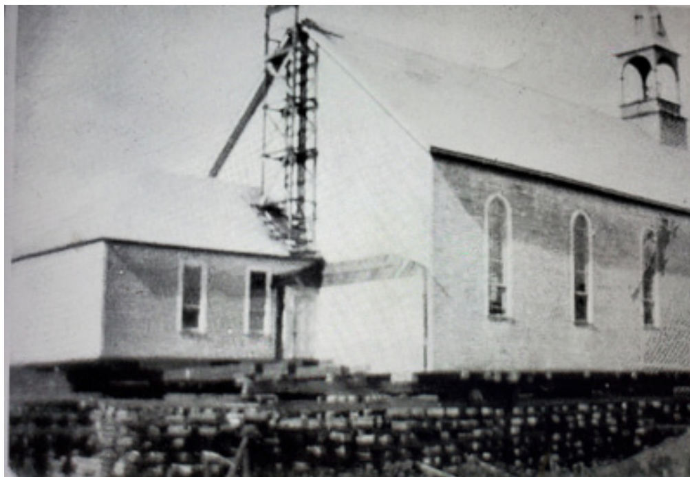
Figure 126 SHVG (s.d.) Images of the original church which was moved as the land was flooded when the Pagan Dam in Low was built
